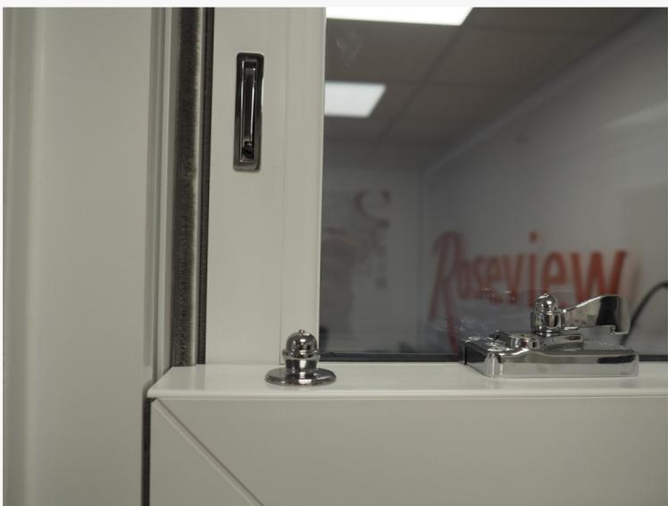
Normally the limit stops will be in the “out” position, which prevents the sashes from sliding more than around 100mm (4 inches)
