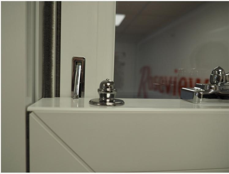
Your windows may be fitted with limit stops (called “shark fins”), which restrict the amount that the top and bottom sashes can open to around 100mm (4 inches). These can be temporarily closed to allow your windows to open more.
