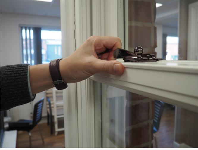
Operating your sash windows is extremely simple. Just unlock the window and then slide the bottom sash up and/or the top sash down as required.
