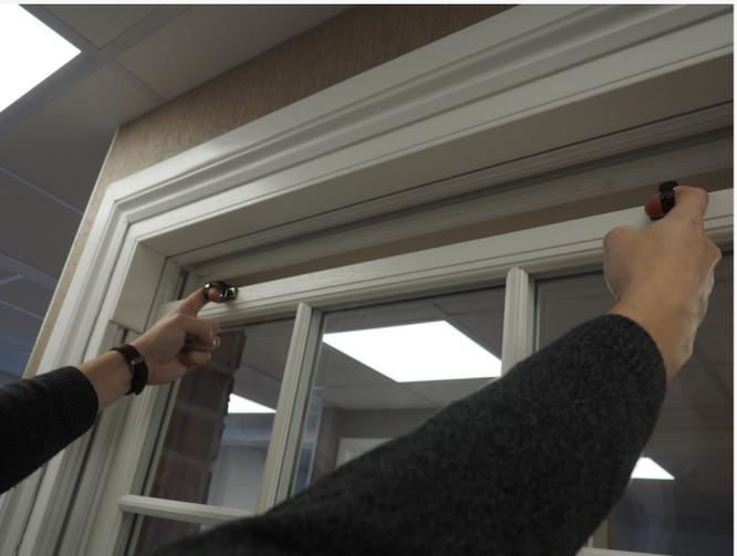
To open the bottom sash, raise the sash using the lift handles. To open the top sash, lower the sash using the ring pull handle.
